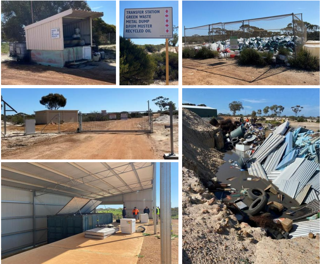
Figure 2.2 Pingrup Refuse Site infrastructure
