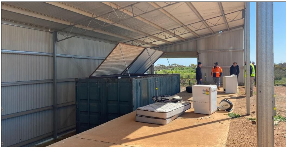
Figure 3.1 Pingrup Transfer Station Shed
