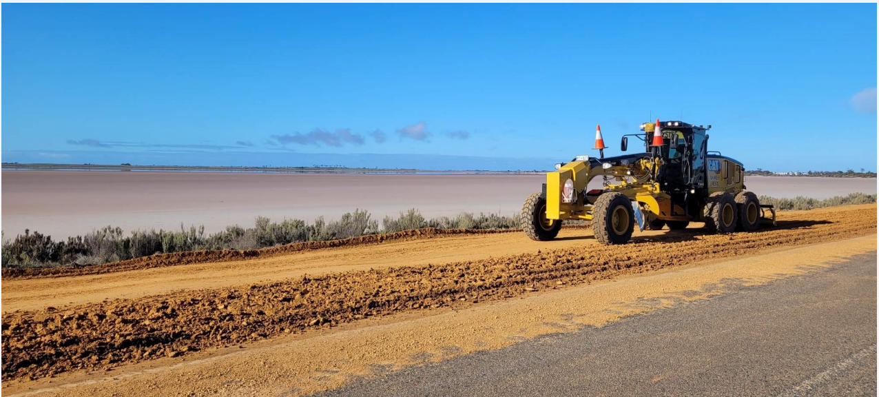
Construction of Ongerup-Pingrup Rd Pull Over Bay
