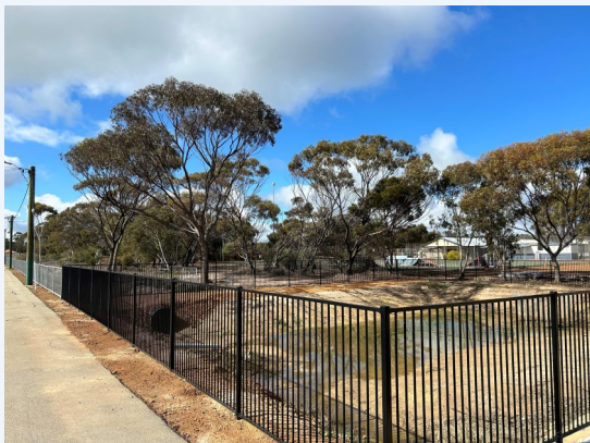
New Fence at Miller's Pond
